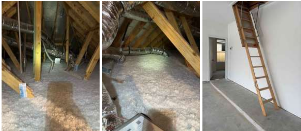
Attic access is in garage
