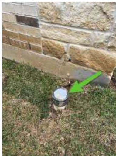
Main drain cleanout is left side of home
