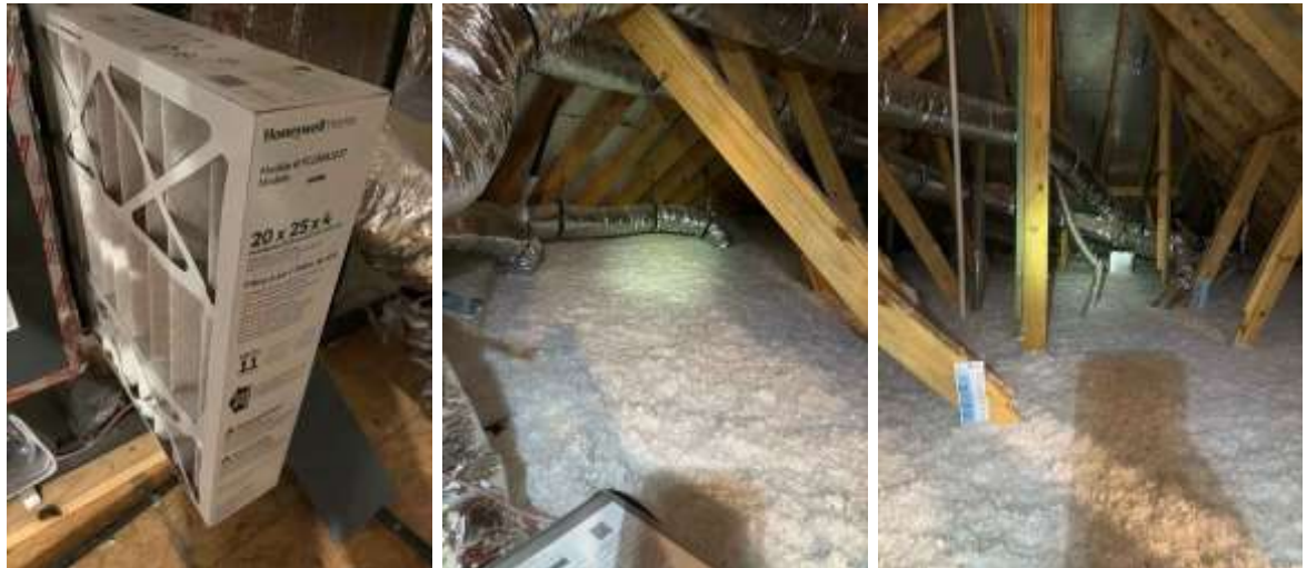
20 x 25 x 4 HVAC filter size
